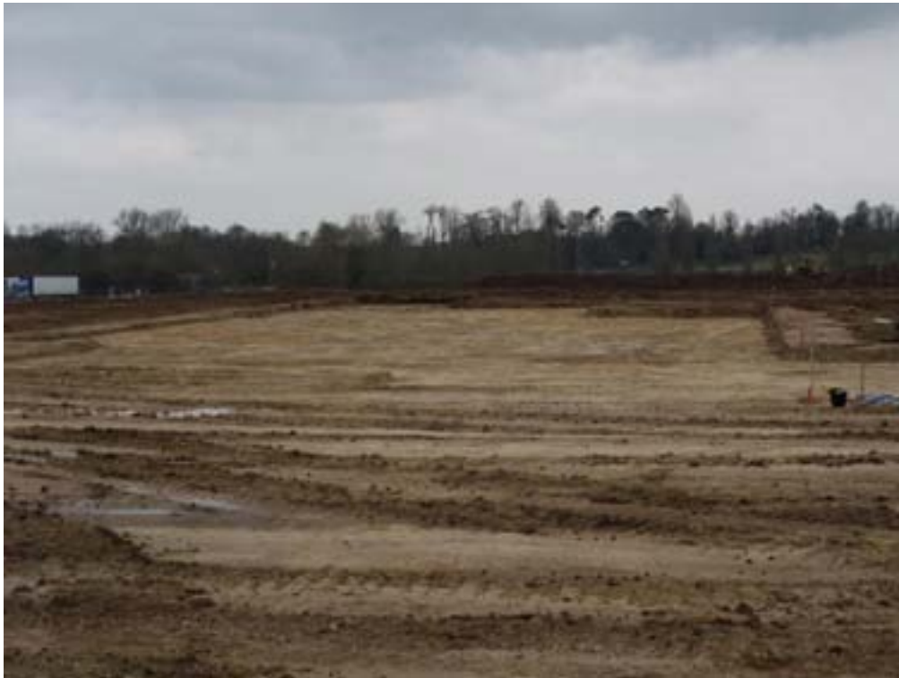
Clubhouse footprint cut out
